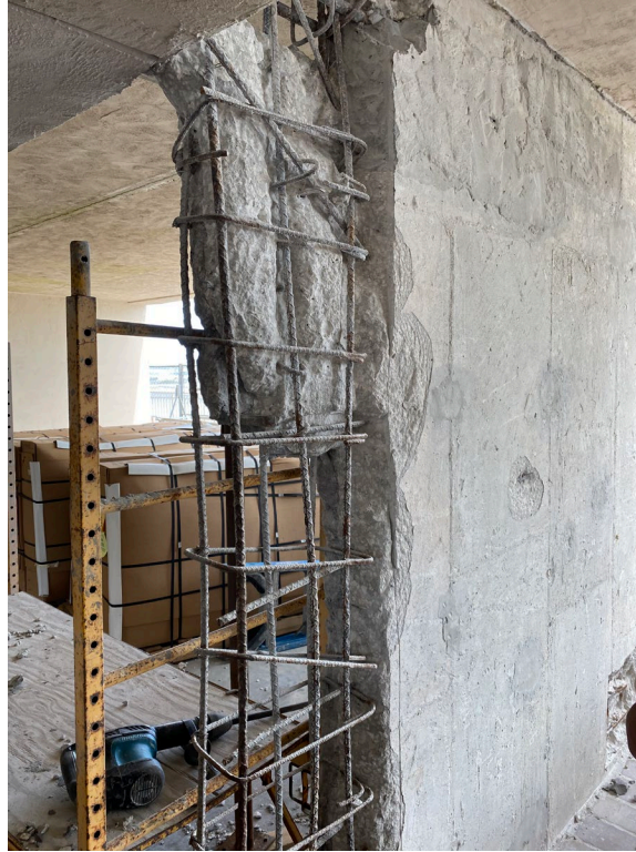
Picture 1: In-progress concrete demo
