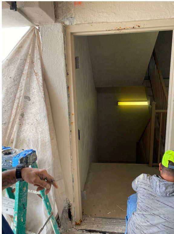
Picture 4: In-progress stairwell door removal
