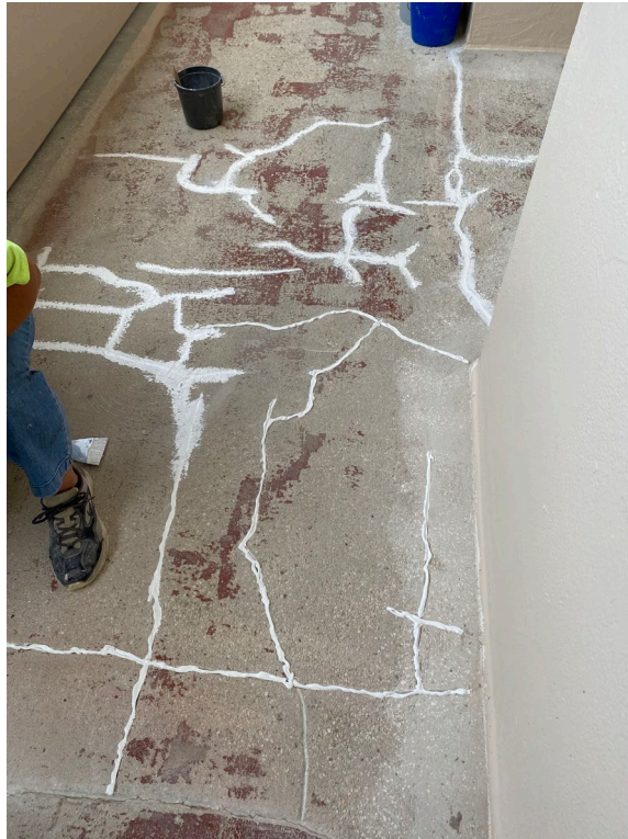
Picture 3: In-progress routing and sealing
