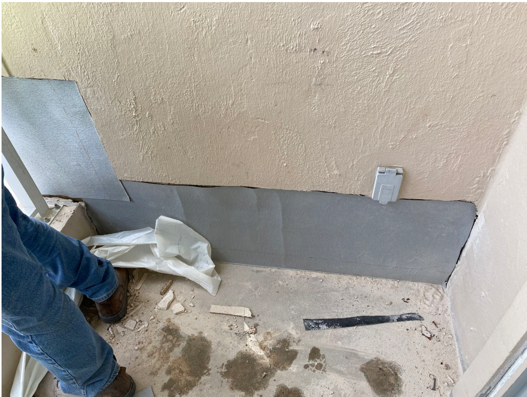
Picture 2: In-progress stucco repair on balcony
